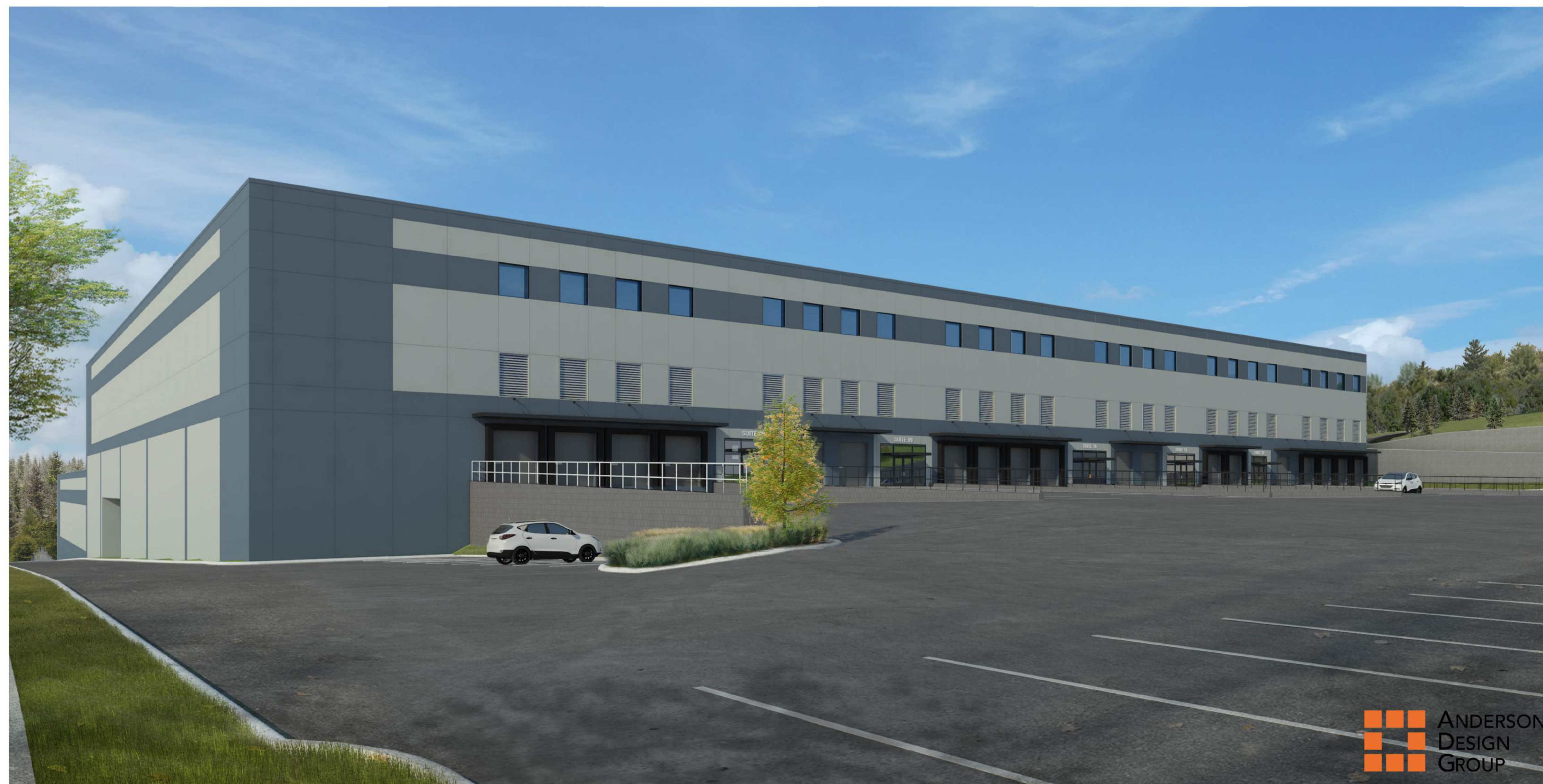
② SOUTH-WEST EXTERIOR VIEW
